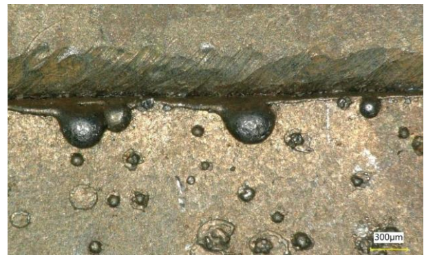
Figure 8 Linear misalignment forming a crevice and spatter on inner surface of pipe in branch A
