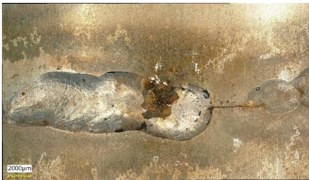
Figure 7 Lack of fusion in the weld root and corrosion spot indicating attack of weld metal, pipe in branch B
