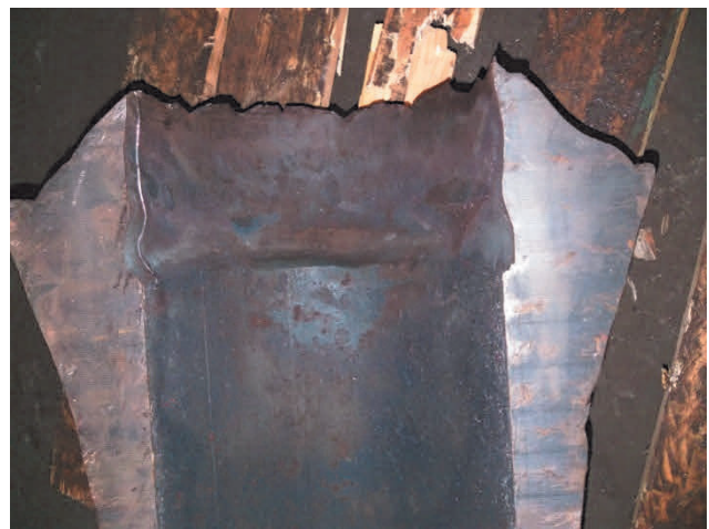
Figure 4 The part of the pipe bell after rolling in a pilgrim mill with changed settings of the rolls of the rolling mill
