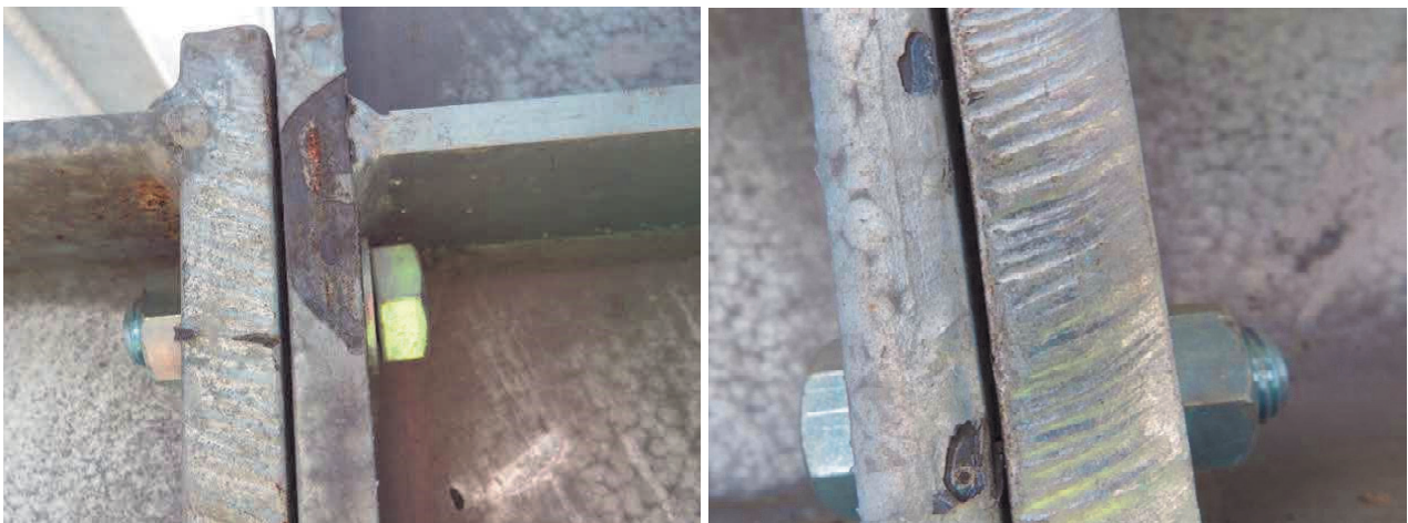
Figure 2 The example of zinc coating on cut edges
