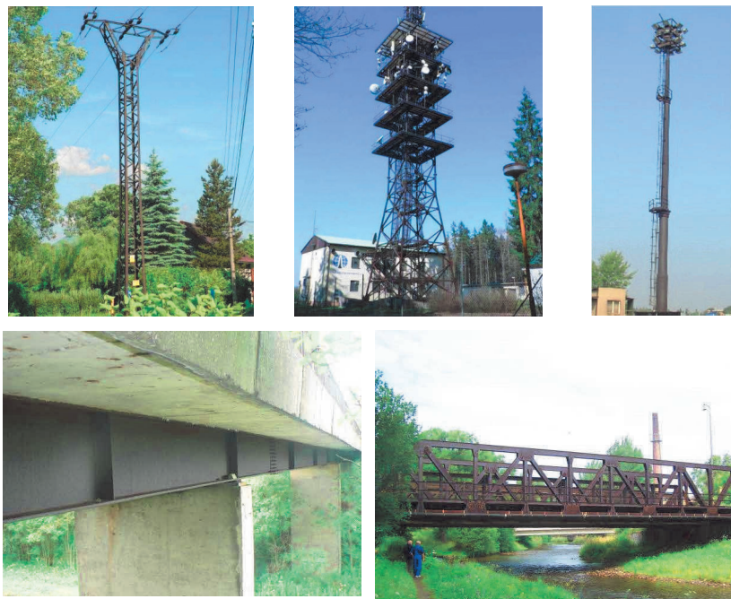
Figure 1 Examples of steel structures built in 1970ties from weathering steel
