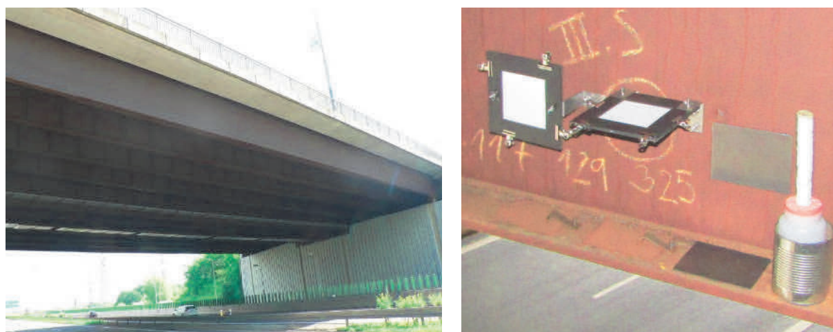
Figure 5 Views of a tested bridge structure
