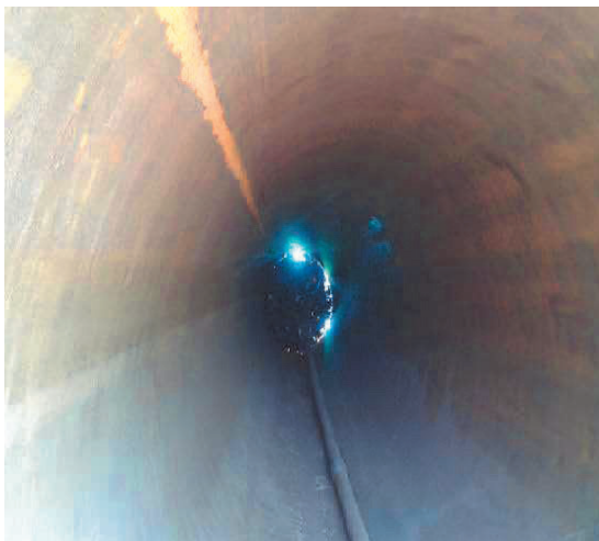
Figure 3 Internal welding of the root pass using 3 welding heads simultaneously
