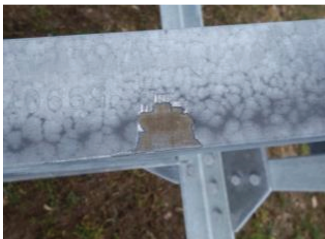
Figure 1 Example of delamination of HDG coating on construction's elements
